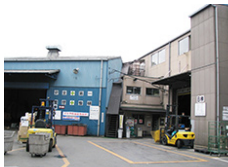
Shikahama Recycling Center, KANAME KOGYO Co., Ltd.
