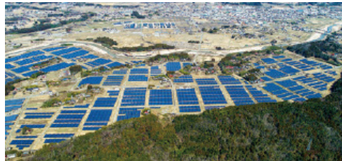
Namie Sakai Solar Power Plant 1 and 2 in Namie Town, Fukushima Prefecture, Japan
