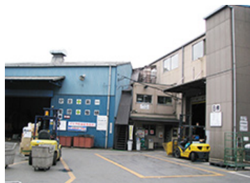
Shikahama Recycling Center, KANAME KOGYO Co., Ltd.
