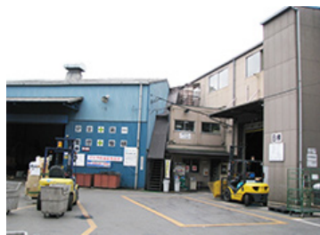
Shikahama Recycling Center, KANAME KOGYO Co., Ltd.
