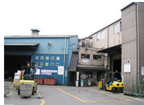
Shikahama Recycling Center, KANAME KOGYO Co., Ltd.
