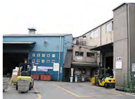
Shikahama Recycling Center, KANAME KOGYO Co., Ltd.
