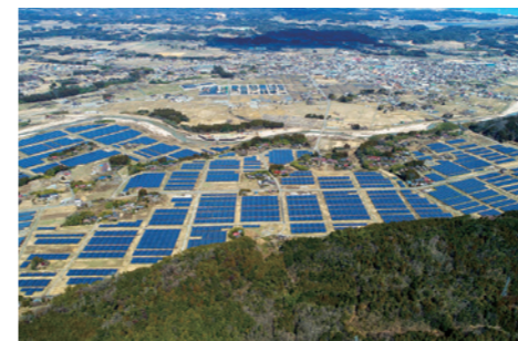
Namie Sakai Solar Power Plant 1 and 2 (Fukushima, Namie) (2020)
